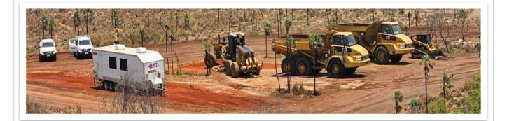
The foundation works in the crossing have now been completed with RTL taking delivery of the corrugated steel pipes which will be used as the culverts. When completed the culvert designs main purpose will be to allow for wet season flooding to pass through the central culvert with the intention of also allowing fish to migrate up and down the creek. The culvert will remain in place for the term of the project.
